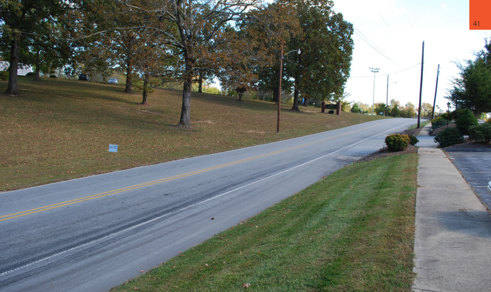
GROVE STREET — EXISTING
