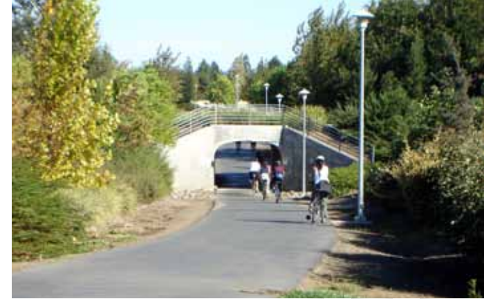
Type 3 crossings (like this crossing in Davis, CA) are grade separated - over or under the roadway - and segregate trail users from motorized traffic completely. Type 3 are recommended on higher speed/higher volume roadways.
