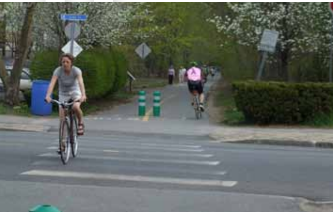
Type 1 crossings (like this crossing of the Springwater Trail in Portland, OR) are used on lower speed, lower volume roadways. Type 1 do not have traffic signals but should include other traffic control devices, such as a clearly marked crosswalk (ladder style is most visible), warning signs, curb extensions, or pedestrian refuges.
