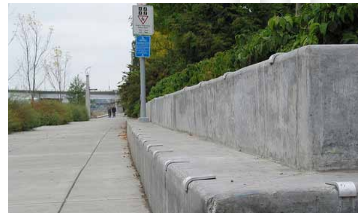
Retaining wall doubles as seating
