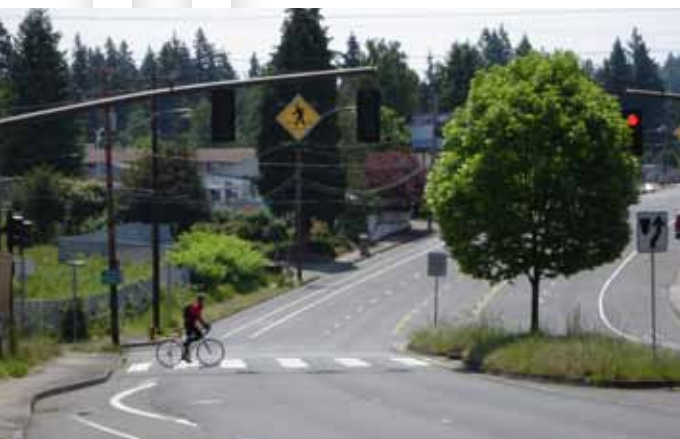
Type 2 crossings (like this crossing of the Springwater Trail in Portland, OR) are recommended on higher speed/higher volume roadways. They are signalized and may include other traffic control devices such as a clearly marked crosswalk (ladder style is most visible), warning signs, and possibly curb extensions and pedestrian refuges.
