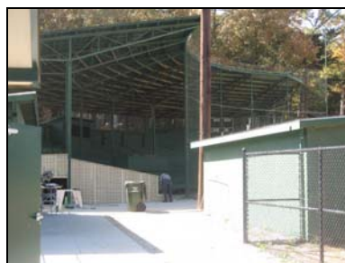
Existing ball field grandstand.
